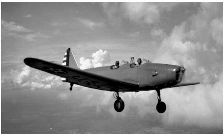
The Fairchild PT-19, with its mono-wing construction most closely resembled the aircraft cadets would graduate to and fly operationally. (USAAF photo from the AAHS photo archives, AAHS-6270)
